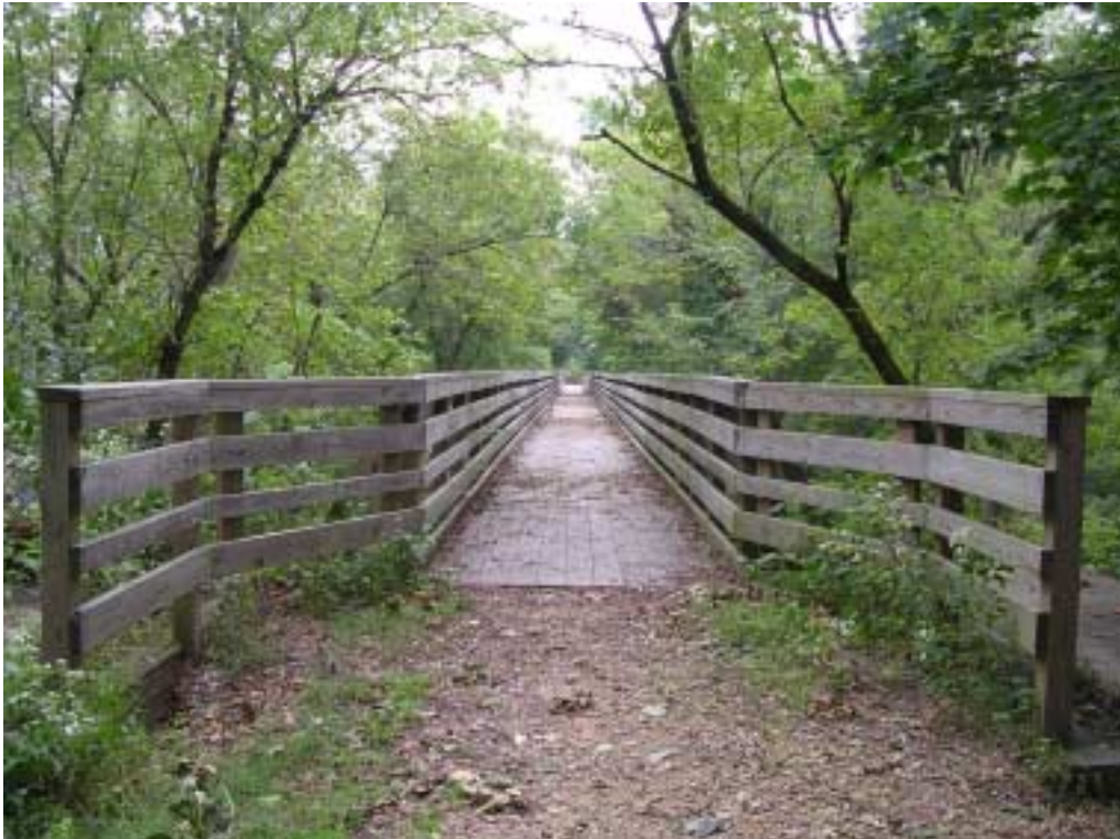
Railroad Bridge on spur of Wissahickon Green Ribbon Trail.
